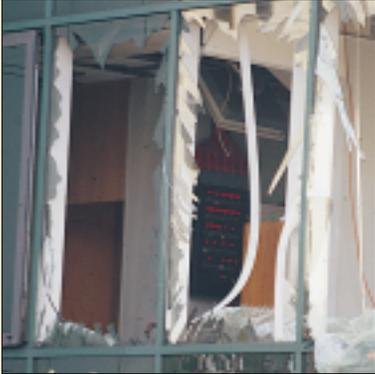
**Glass without a daylight application of security window film is blown out of the frame producing lethal cutting shards on breaking.**
